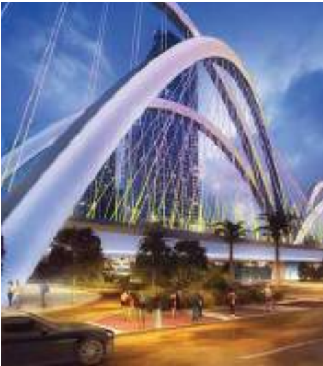
I-395 Bridge & Under Deck Park
